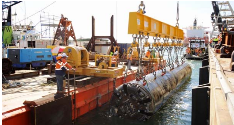
Recovery of TBM from the sea.
