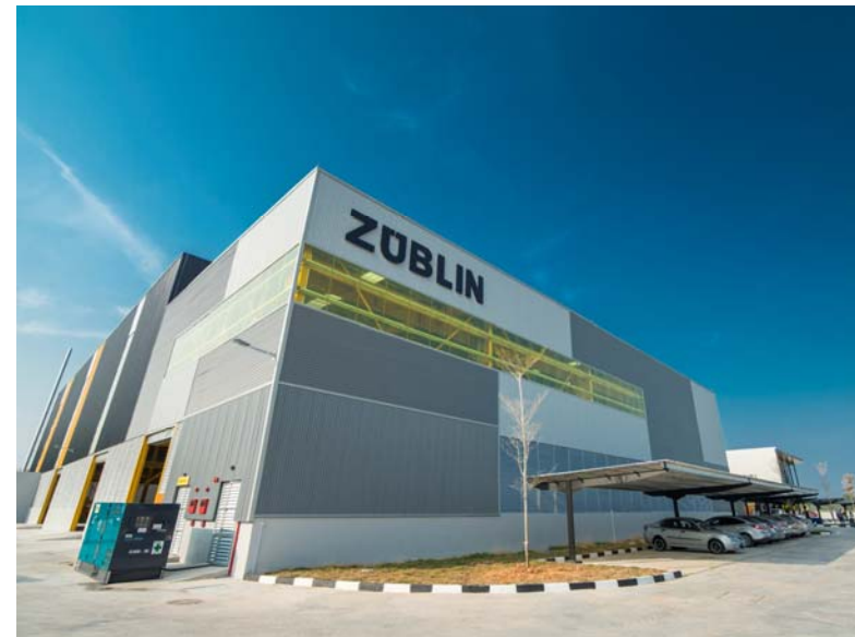
ZÜBLIN Precast Industries Sdn. Bhd. in Johor, Malaysia.
